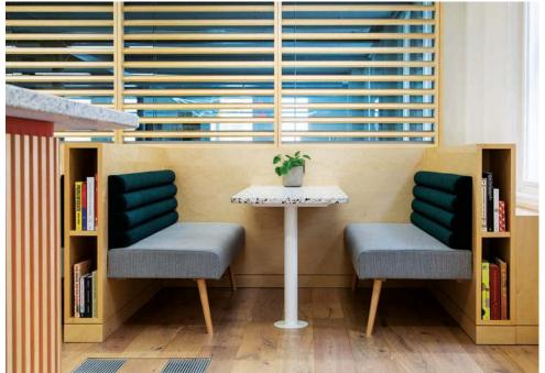
Louvred, slatted screens were incorporated into these seating booths, manufactured from birch veneered plywood.
