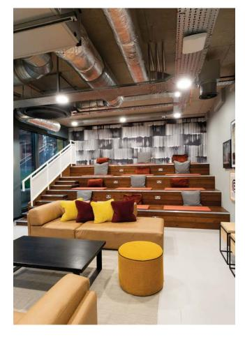
Stained softwood with aluminium nosings, are used to form the external fascia panels of this bleacher seating.
