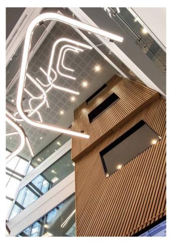
Horizontal, vertical and diagonal slats of oak are used to clad this large atrium wall, pierced by a series of viewing apertures.
